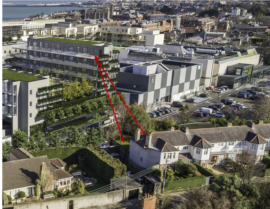
Aerial view of the south east corner of the previous pre planning scheme highlighting potential impact on the adjoining houses in Frascati Park.
